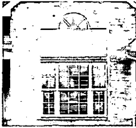
19. Oversized window(s) (larger than minimum building code requirement).
