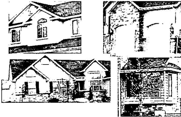
27. Cantilevers "Pop Outs" and setbacks to different parts of the home that break up otherwise long uninterrupted wall planes.
