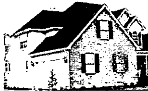
11. Side entry garage with windows in the exterior garage wall that faces the front yard.
