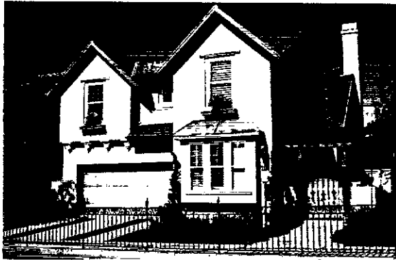
Main gable roof with intersecting gable roofs
