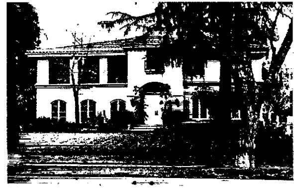
Belt course trim and arched windows
