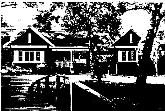
Simple massing and gabled roof forms
