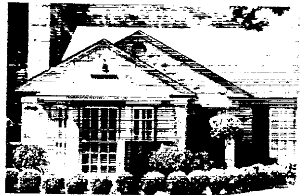
Broken pediment and vents at gables, bay window, shutters
