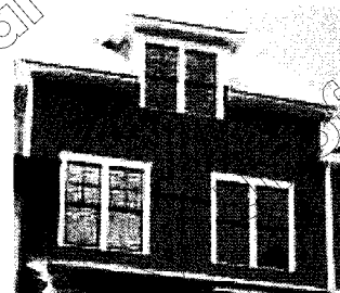
Shutters not prominent in Park Homes
