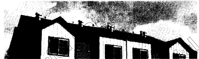
Mechanical vents reflect architectural style
