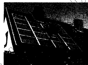
Solar panels visual impacts are minimized
