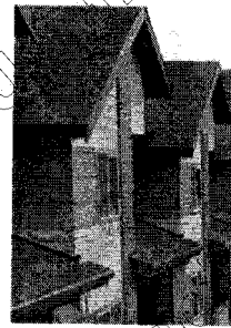
Overhangs protect walls
