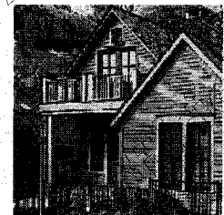
Porch roof breaks up two story element
