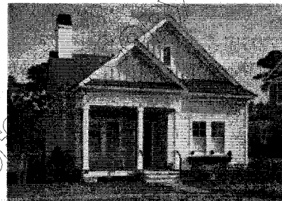
Porch roof forms are consistent with home
