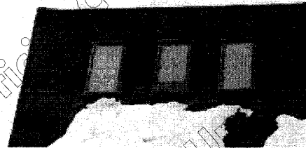
Skylights are flat to roof and do not extend to eavelines or roof peaks
