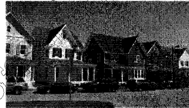
Not this - Similar two-story homes repeated too often
