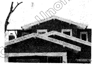
Appropriate roof overhangs
