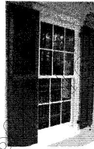
Shutters sized to match openings
