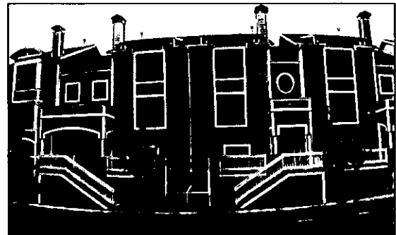
Townhouse development Utah County
