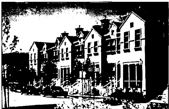
Townhouse development Utah County
