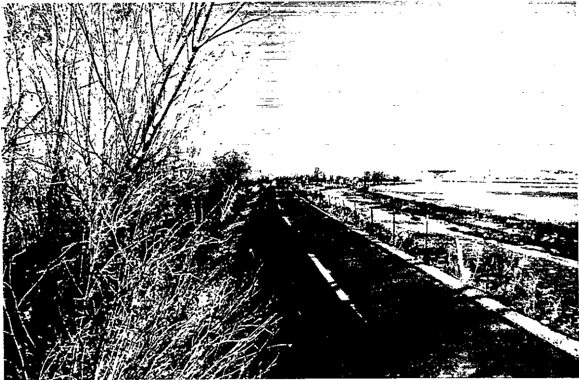
Dike/trail looking North, canal is on the right of the photo.
