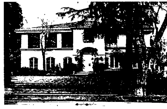
Belt course trim and arched windows
