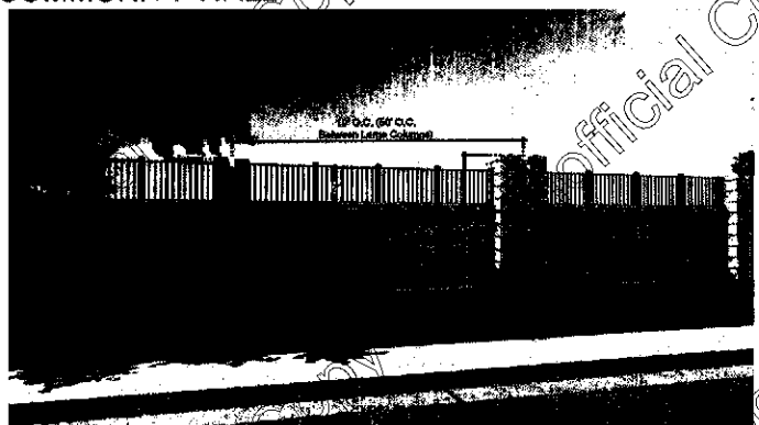
VIEW WALL - PARTIAL
