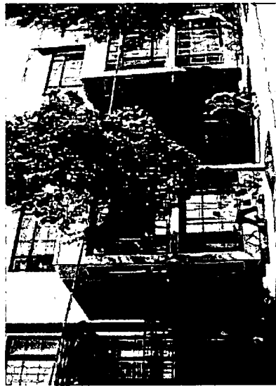
These townhomes incorporate off-street parking within the structure.
