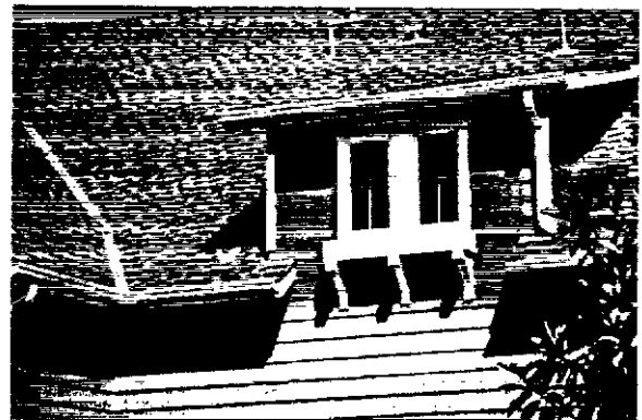
Shed roof dormer and flower box detail
