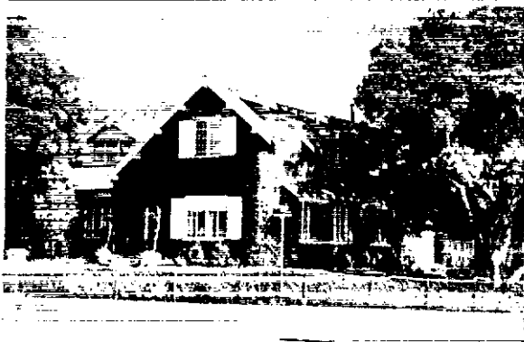
Front to back roof with intersecting shed roof
