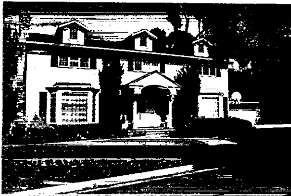
Covered entry with wood columns
