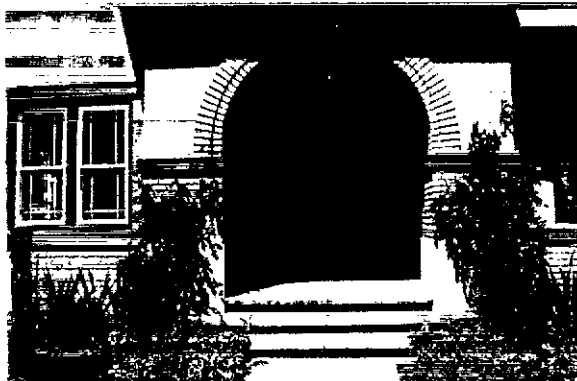
Brick accent at entry alcove
