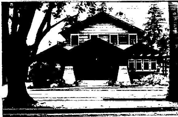
Simple gabled roofs and battered porch columns
