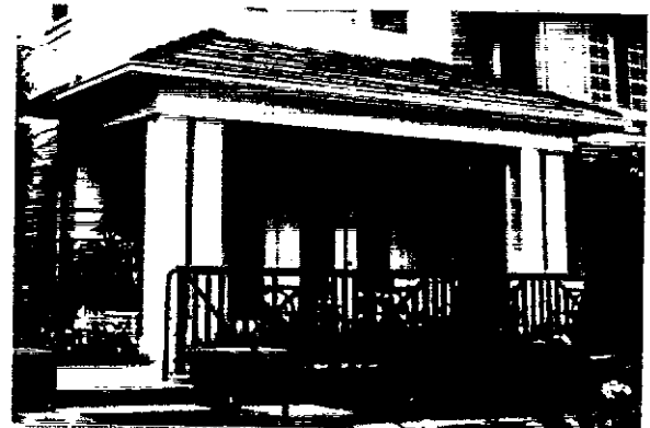
Squared wood-like columns with trim
