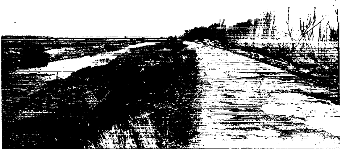
West airport dike looking southward, the ground-water collection canal is located on the inward side of the dike
