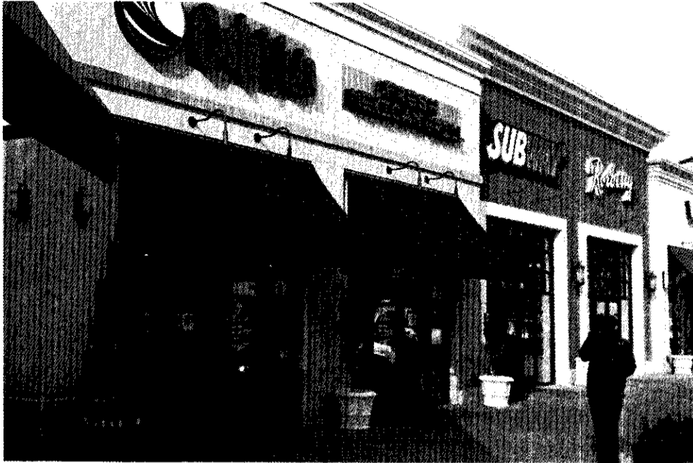
Awnings provide a more inviting entrance. Cornicing on top adds style and character.
