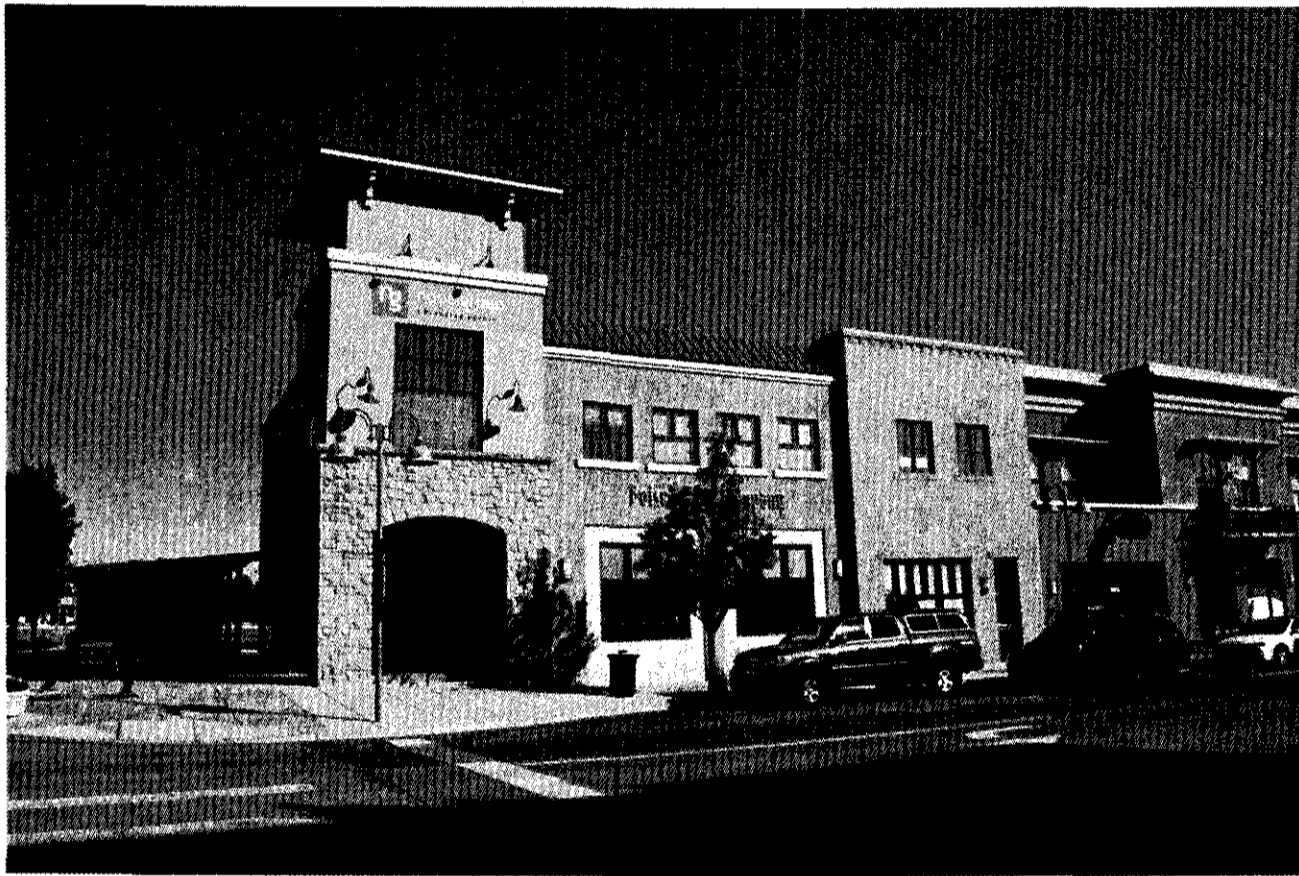
Unique corner architectural design at entrance to site.
