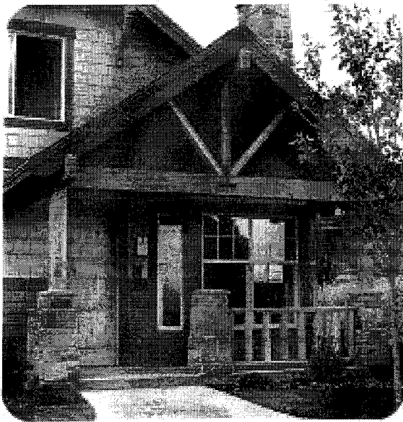
Mixed use of stone, siding, and timbers.
