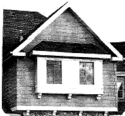
Shingle siding, window pop out, and decorative corbels.
