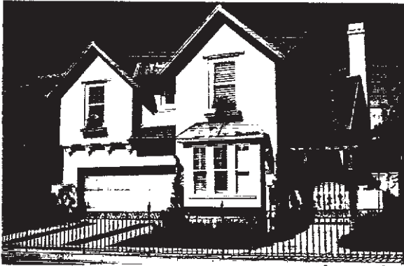
Main gable roof with intersecting gable roofs
