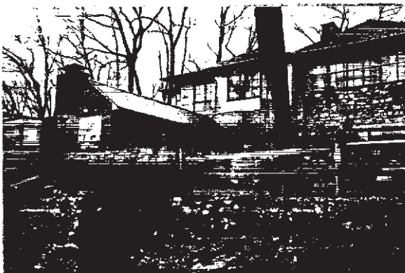
Primarily hip and gable roof elements
