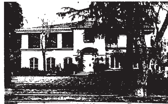
Belt course trim and arched windows
