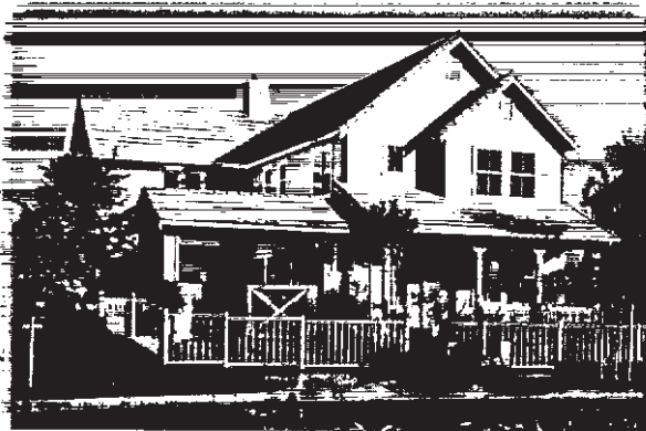
Fully wrapped siding
