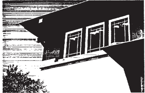
Belt course trim and boxed soffit
