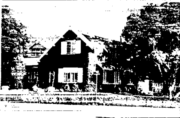
Front to back roof with intersecting shed roof
