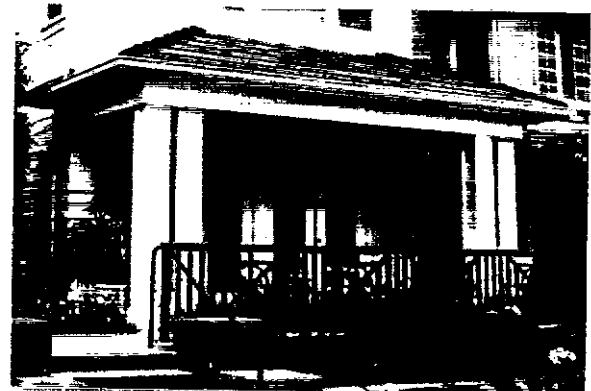
Squared wood-like columns with trim
