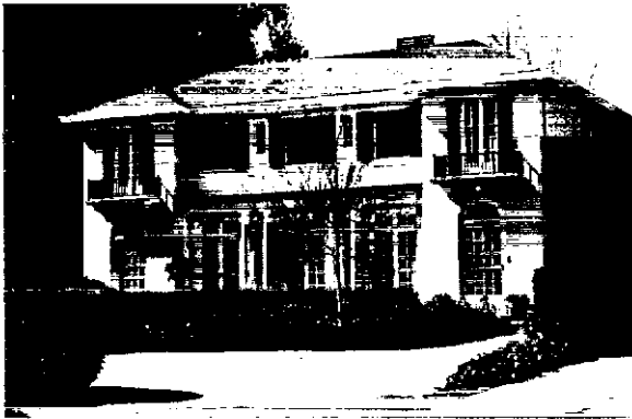
Main hip roof with minor intersecting hip roofs
