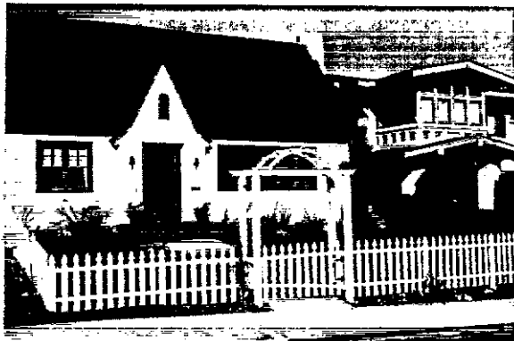
Entry roof form
