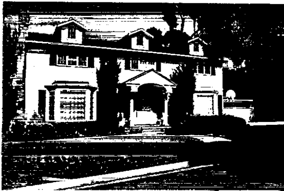
Covered entry with wood columns
