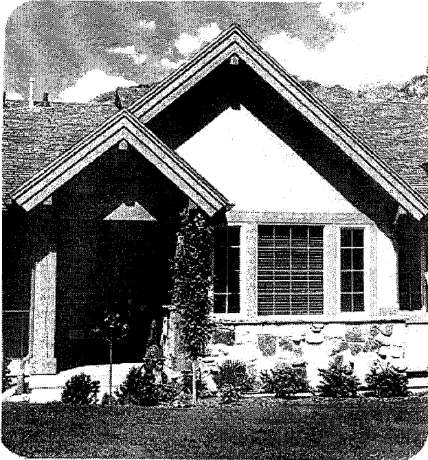
Stone wainscot and stucco with roughsawn timbers as structural support for the porch roof.
