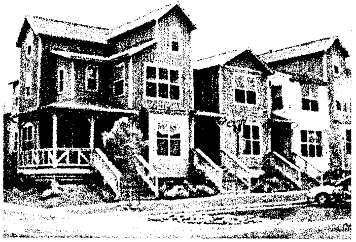
A well-articulated corner treatment with wrapped porch addressing both streets. Miller Ranch, Edwards, Colorado.
