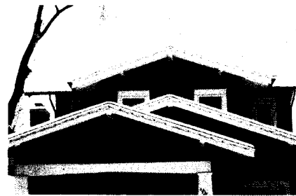
Appropriate roof overhangs
