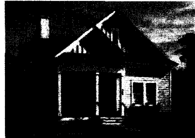
Porch roof forms are consistent with home
