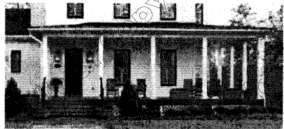
Porch raised above finished grade
