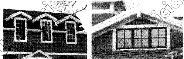
Window heads must be level
