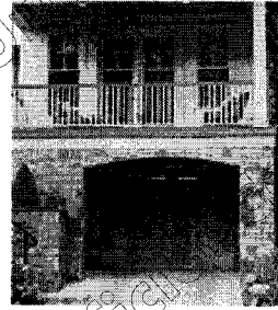
Patio over garage lessens its visual impact
