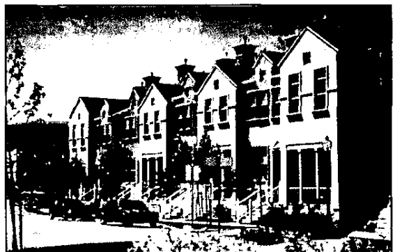
Townhouse development Utah County
