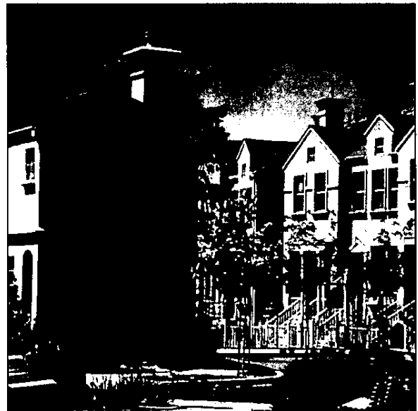
Two story apartment complex
