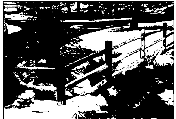
Example wood fencing
