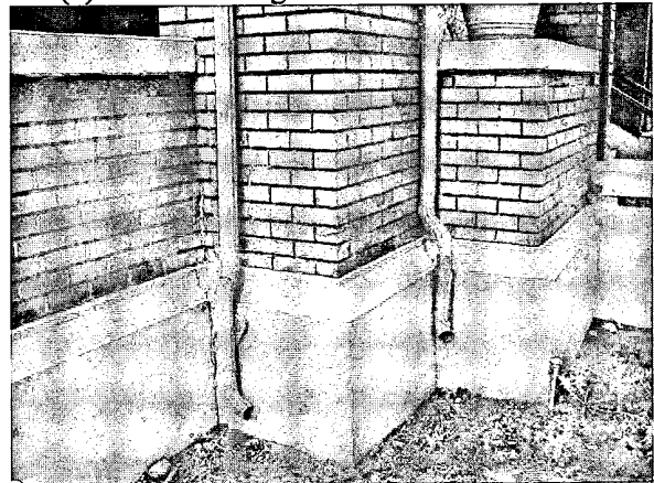
(6) Water staining to brick
