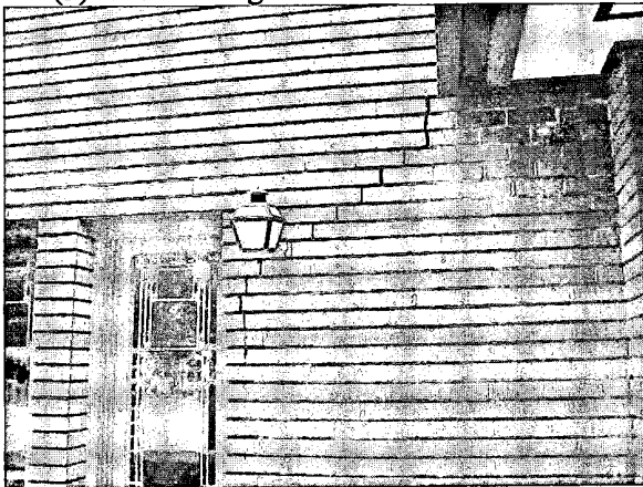
(3) Crack through brick west of French doors
