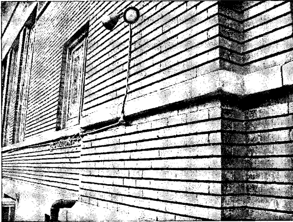
(9) Crack in foundation
