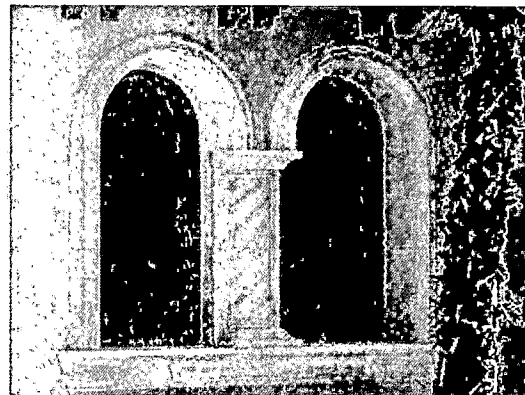
Not Allowed – Arch Windows
