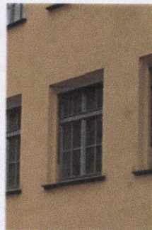
PERMITTED: thick stucco for deep relief
