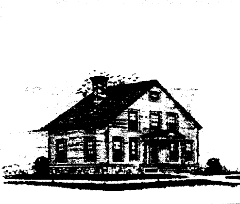
VIEW BEFORE ALTERATION.
