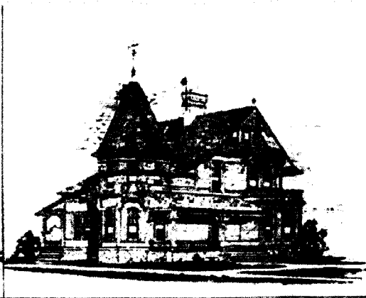
VIEW AFTER ALTERATION.
