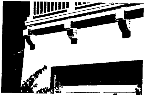
Shaped corbels and recessed garage door
