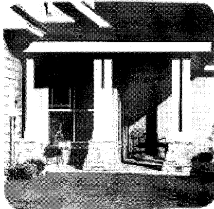
Stone accent base on wood roof supports.
